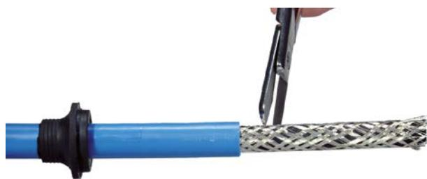
Cut the shield 1cm from the cable sheath
